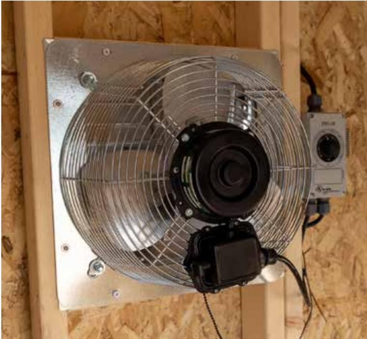
Louvered Fan w/ Power Shutter & Thermostat
